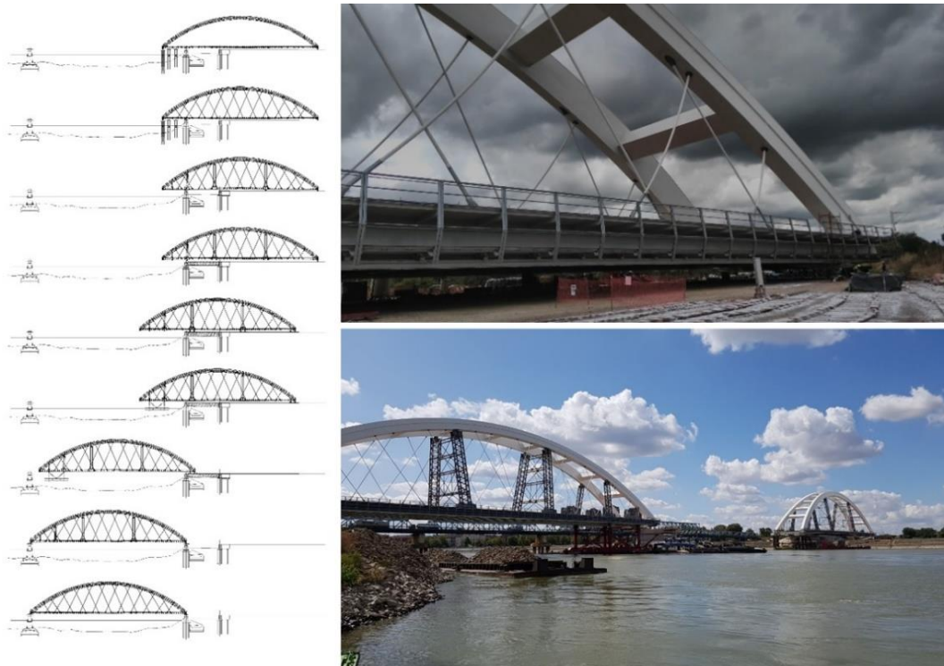
Figure 9. Launching of arch bridges over the Danube.
